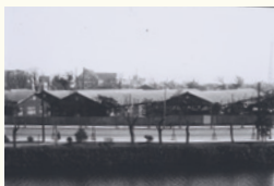
1924(大正13)年、焼失した元衛町の校舎に代わり新築された仮校舎(麹町区竹平町1番地) 1924: The temporary school building was built to replace the school building in Motoe-cho, which was destroyed by fire (1 Takehira-cho, Kojimachi-ku, Tokyo).
