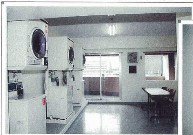
Laundry room (Building 1)
